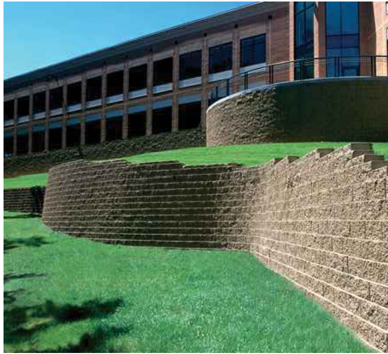
TERRACED RETAINING WALL
